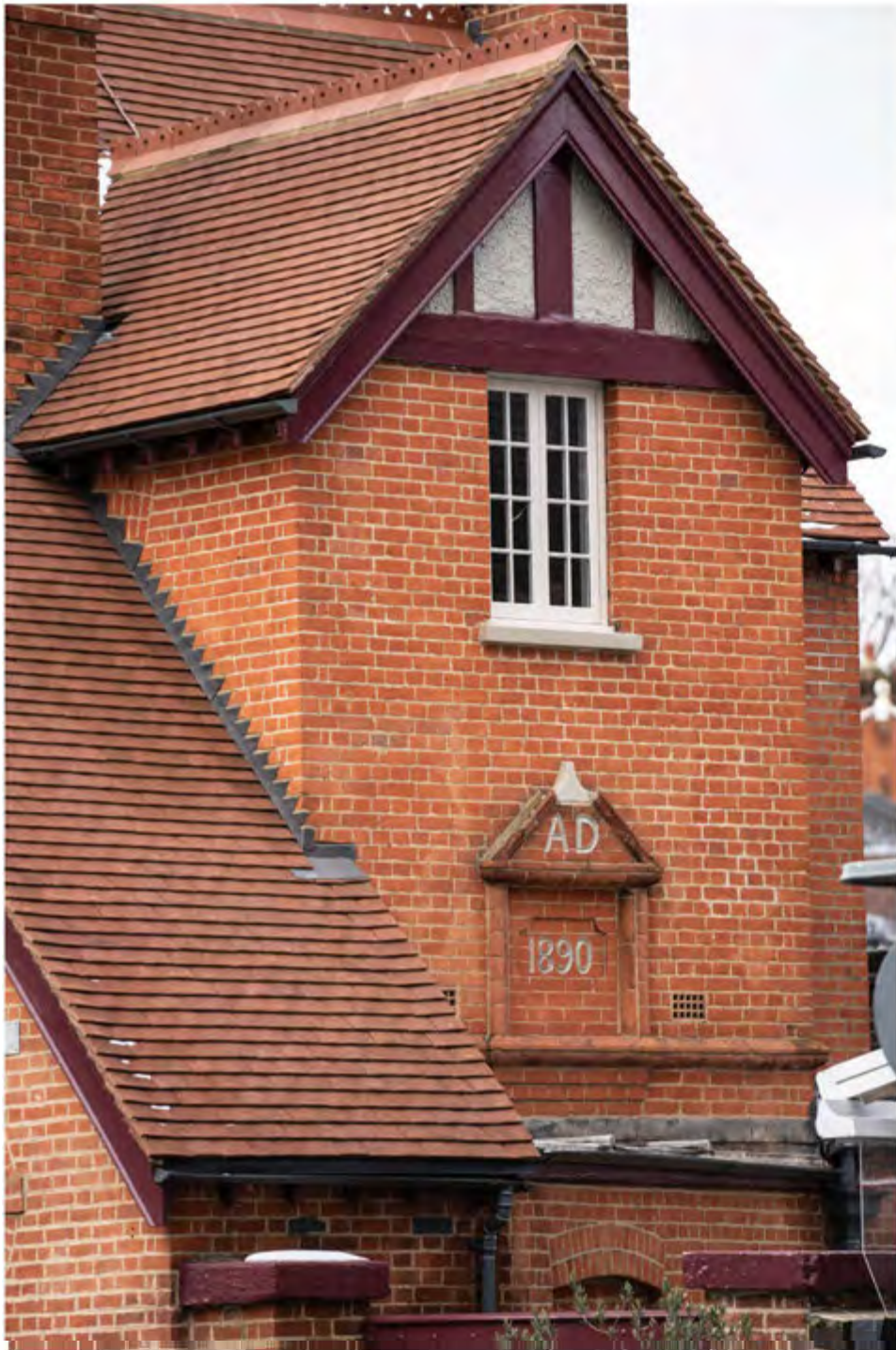
Grade listed 2 building
